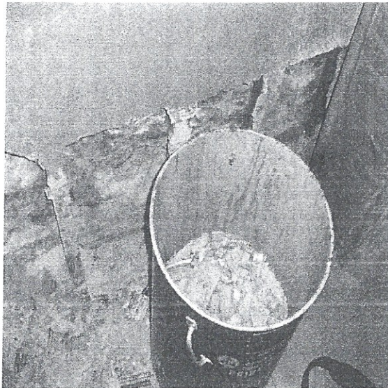
Non-ACM One Coat Plaster and Associated Paint Basement Vault Room
